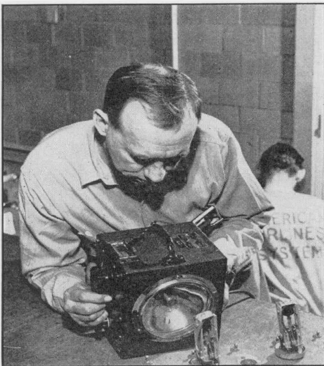
FIGURE 2. The TYPE 631-B Strobotac is used to check vibrator reeds by James Hargreaves, lead mechanic in radio-overhaul shop.
